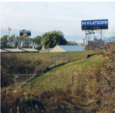
Incompatible foregrounds and backgrounds impact heavily on the image of the fort.
