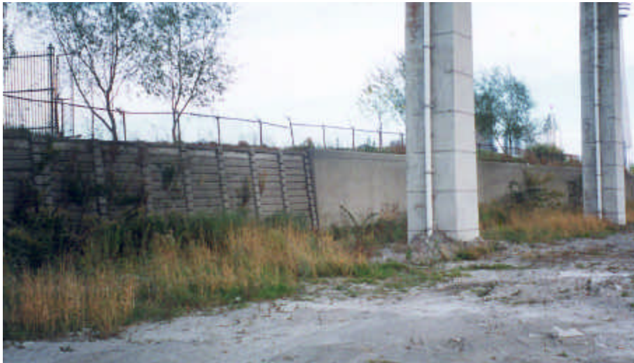
Present view of the retaining walls under the Gardiner Expressway
