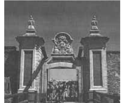
Louisbourg Historical Site Gate Reconstruction
