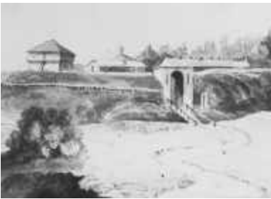
The East Gate to Fort York
