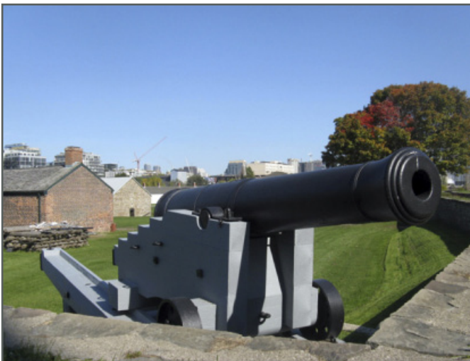
Cast aluminum traversing gun platform and 18 lb gun located at the south-west bastion. (Photo courtesy of Ted Smolak)
