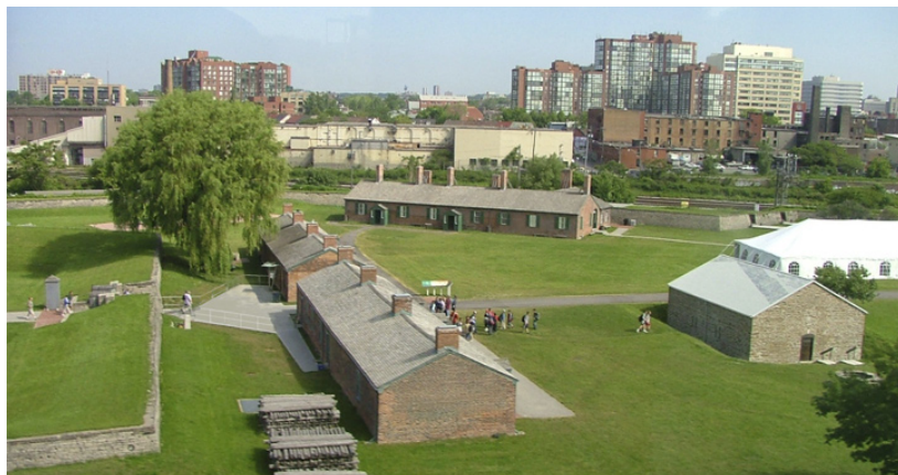
The Thomson family was involved in the 1815 construction of the four brick and stone buildings at the west end of the fort, seen here from the south. The South and North Soldiers' Barracks are to the left, the Officers' Brick Barracks and Mess Establishment in the centre, and the Stone Magazine to the right. (Credit: ntvwebfolio.com)
