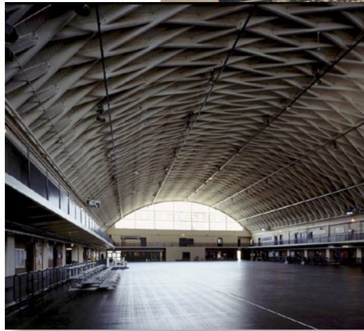
Fort York Armoury under construction, 1934. Canadian Contract Record, 21 Nov. 1934, p989. Interior of armoury with lamella roof. Photo credit: Paul Gauvreau. Both joint-detail sketches also by Paul Gauvreau.
