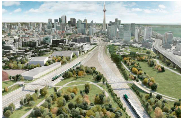
Fort York Pedestrian Bridge looking east toward downtown Toronto. Credit: Image courtesy of DTAH
