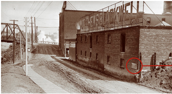
A near identical tablet to the one at the west gate was found at the fort's eastern entrance on the wall of Matthews-Blackwell's pork packing plant. The Canadian Club of Toronto was responsible for having both plaques funded by the Minister of Militia and erected in 1899. The one at the eastern entrance disappeared after the abattoir was demolished in 1929, but not before good photographs in situ had been taken.
