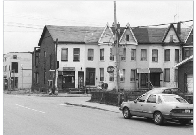
Patrick Cummins, a recorder of Toronto streetscapes par excellence, photographed the buildings from 111 to 117 Niagara on 30 April 1988. The unit at the corner of Tecumseth differed in design to reflect the fact it was intended to be a shop. Credit: Patrick Cummins
