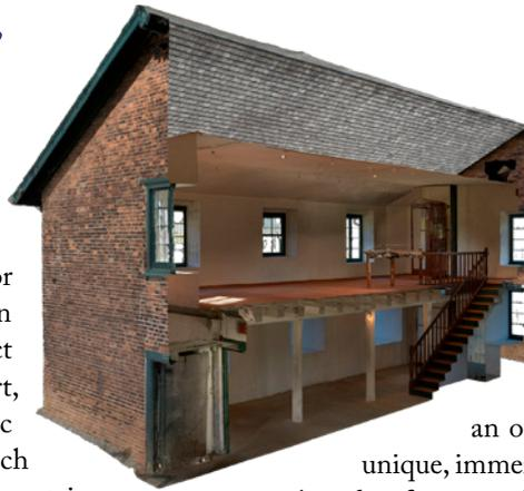
The Brick Magazine in cutaway shows the detail of what the CyArk process can capture. Credit: CyArk and Michael Carter
