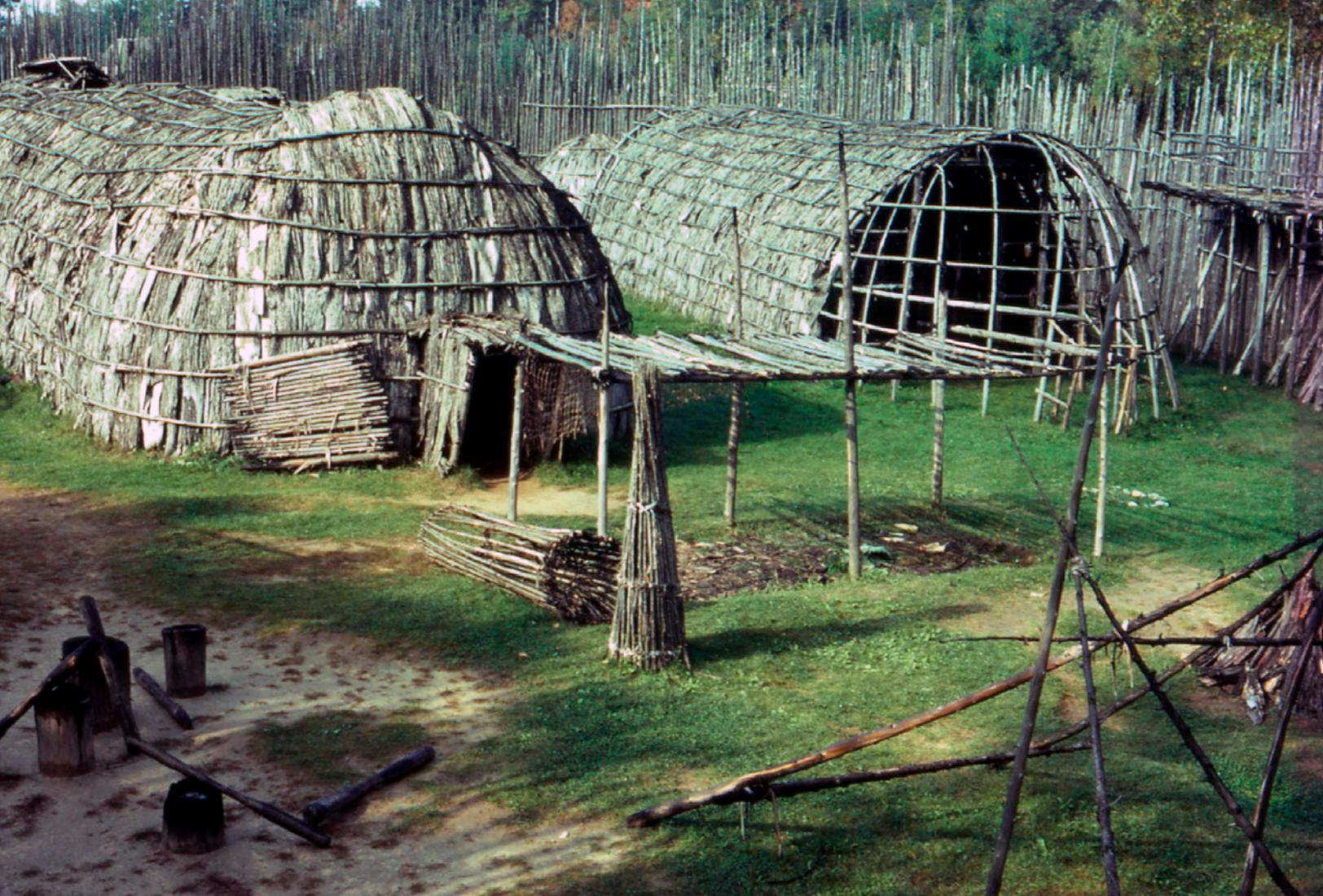
**Wendat longhouses** had a framework of curved poles and were covered with sheets of bark. A series of holes in the roof let light in and the smoke from family hearths out. At left are vessels for pounding corn, while a palisade – with a firing platform at the extreme right – surrounds the village. This reconstruction is *Ska-nah-doh* ('Village stands again') at the Longwoods Conservation Area near London, Ontario. Courtesy Ron Williamson
